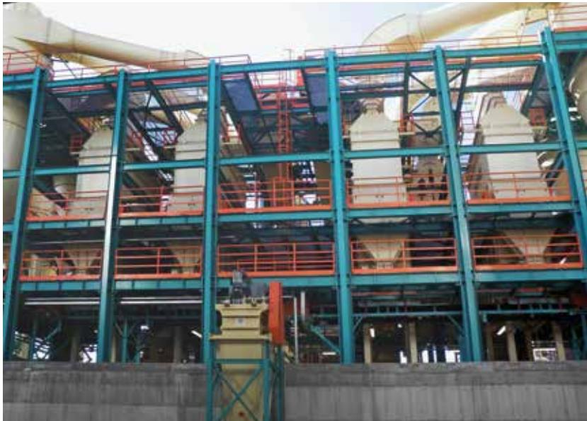
The machine is designed to process particles of wood material in very small fragment form. Using air as a means to separate particles, the machine allows differently sized particles to be separated and, by adjusting the intensity of the air flow, the desired and accepted particles can be separated and conveyed into the cyclone.
